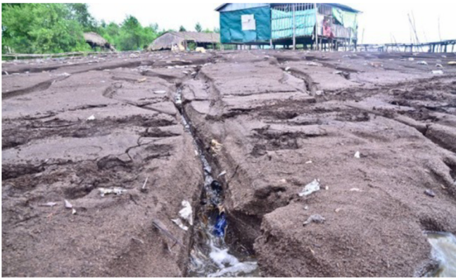
Fig. 5. Erosion and Flooding in Ilaje (Authors, fieldwork, 2017).
